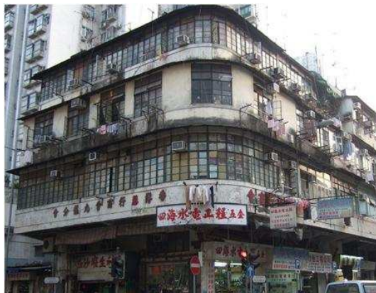
Junction of Pei Ho Street and Hoi Tan Street (2007)
